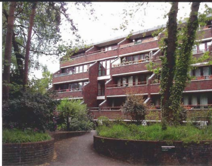
Iveagh Court, Bracknell. Owned by The Guinness Trust. Water-King Sentry water conditioners were chosen to be retro-fitted after extensive trials.
