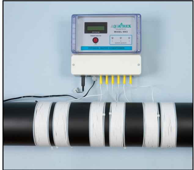
directions from a central point. When facing the pipe, one aerial should start by passing behind the pipe and the other should pass in front of the pipe. Secure each end of the aerial with a cable tie.
